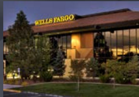
5340 Kietzke Lane, Reno 55,917 SF Class A Office
