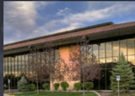
5370 Kietzke Lane, Reno 55,559 SF Class A Office
