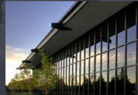
5390 Kietzke Lane, Reno 65,917 SF Class A Office
