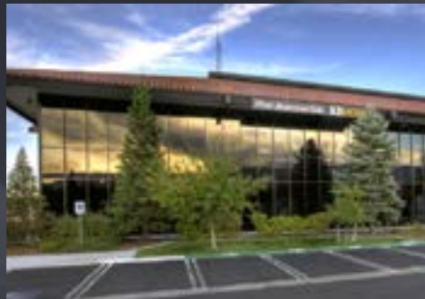
5310 Kietzke Lane, Reno 55,387 SF Class A Office
