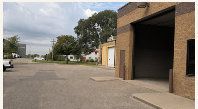
16' wide drive-in door & driveway
