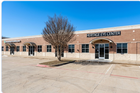
SUBJECT BUILDING Suite 160 entry & signage
