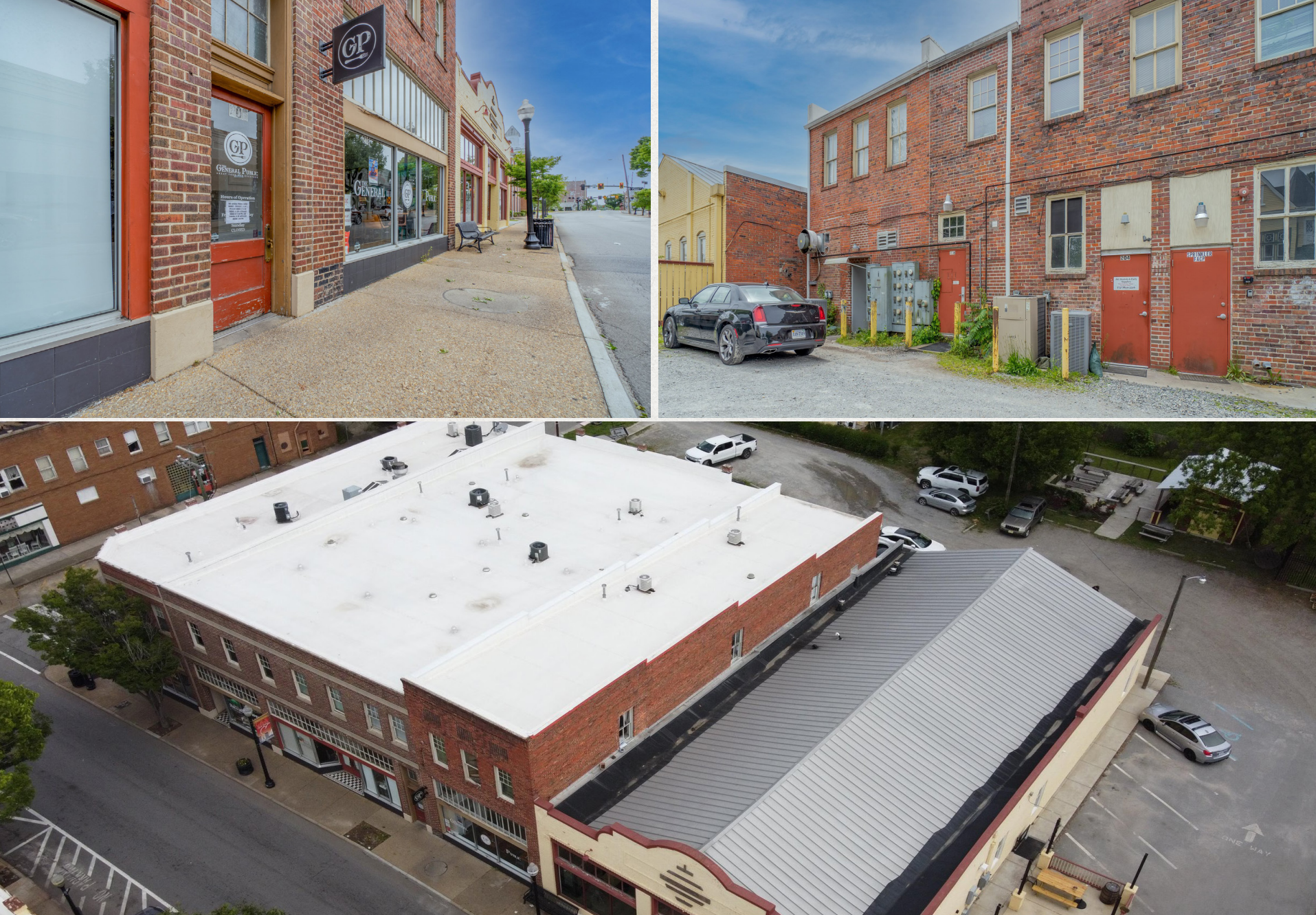
200-208 E WASHINGTON STREET Exterior Photos
