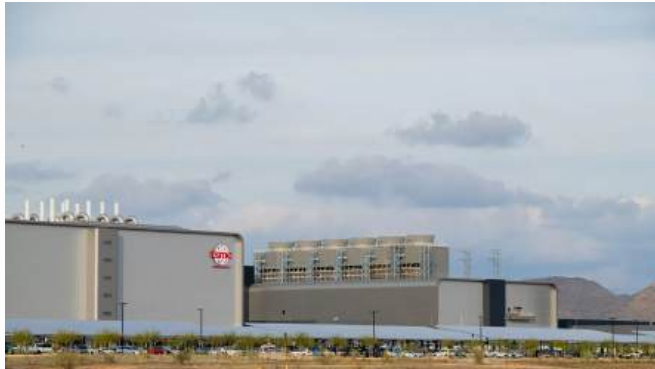
The TSMC facility in Phoenix in 2023.
