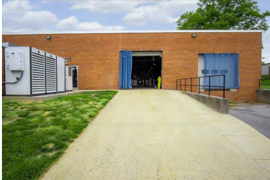
View of Drive In Door
