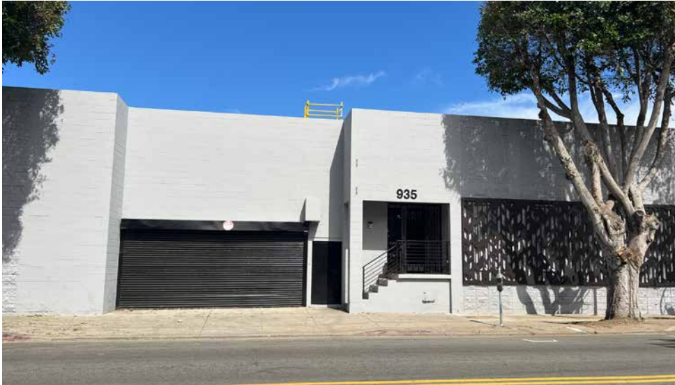
Front of Building
