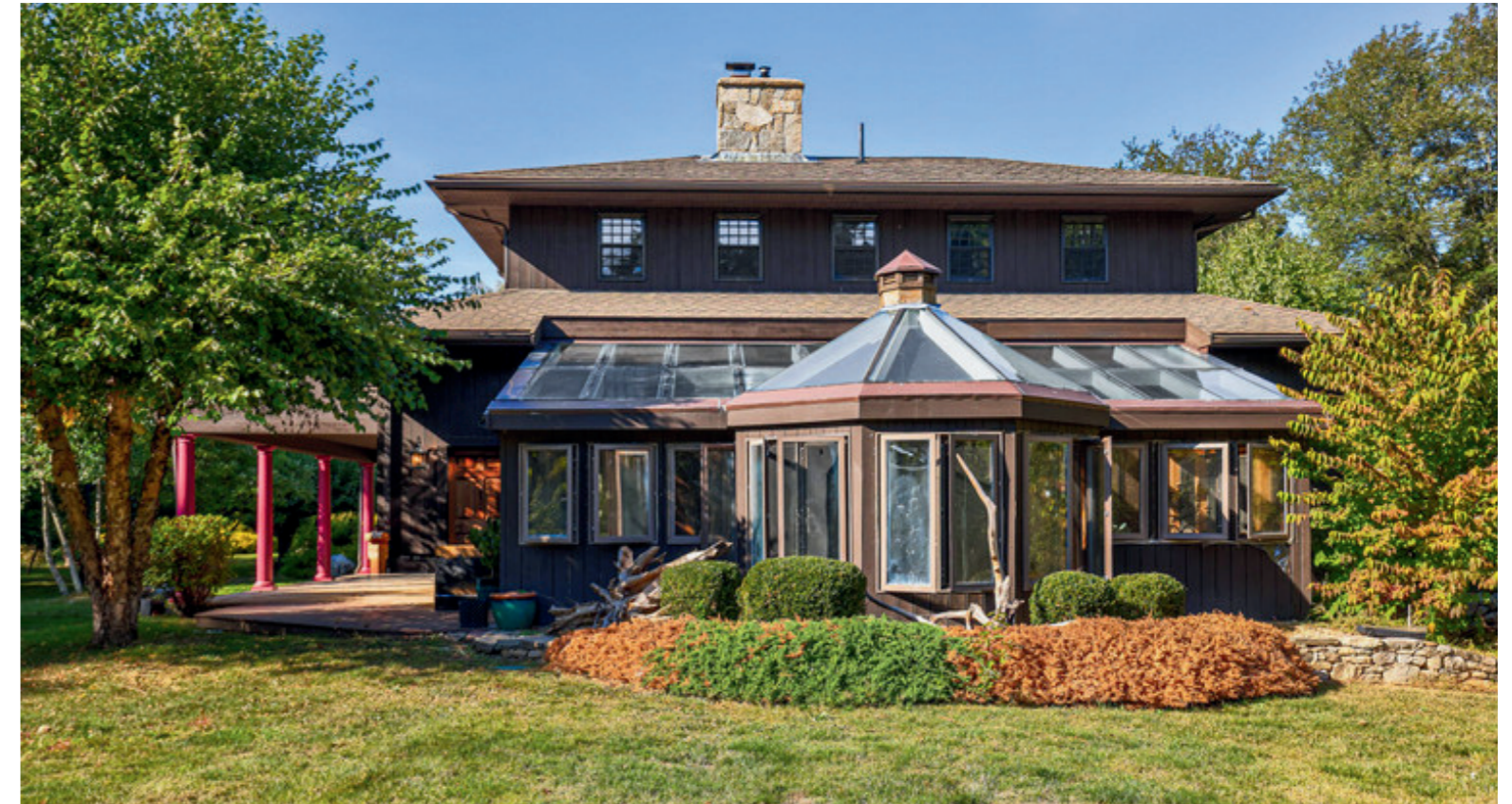
The Caretaker's Cottage
