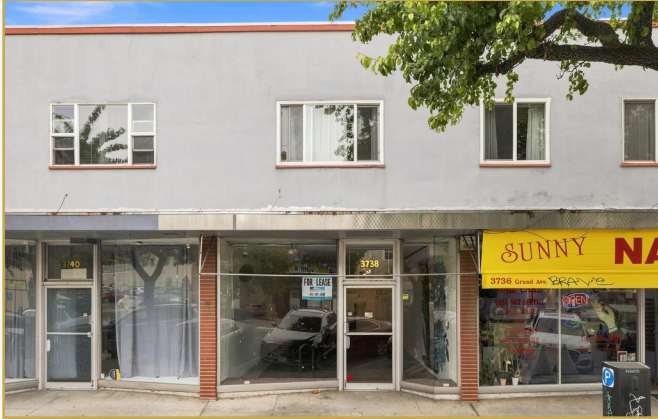
Ground-Floor Commercial Storefronts
