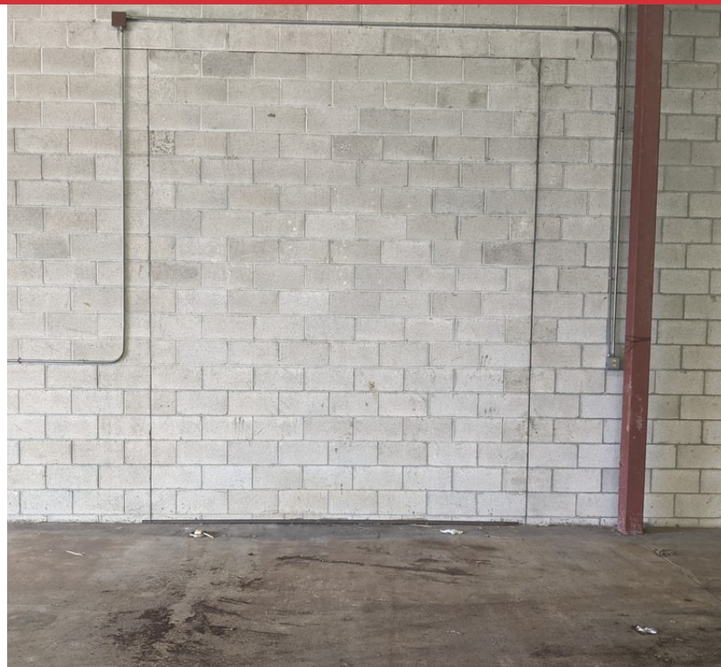
Knock Out Connecting Adjacent Bay
