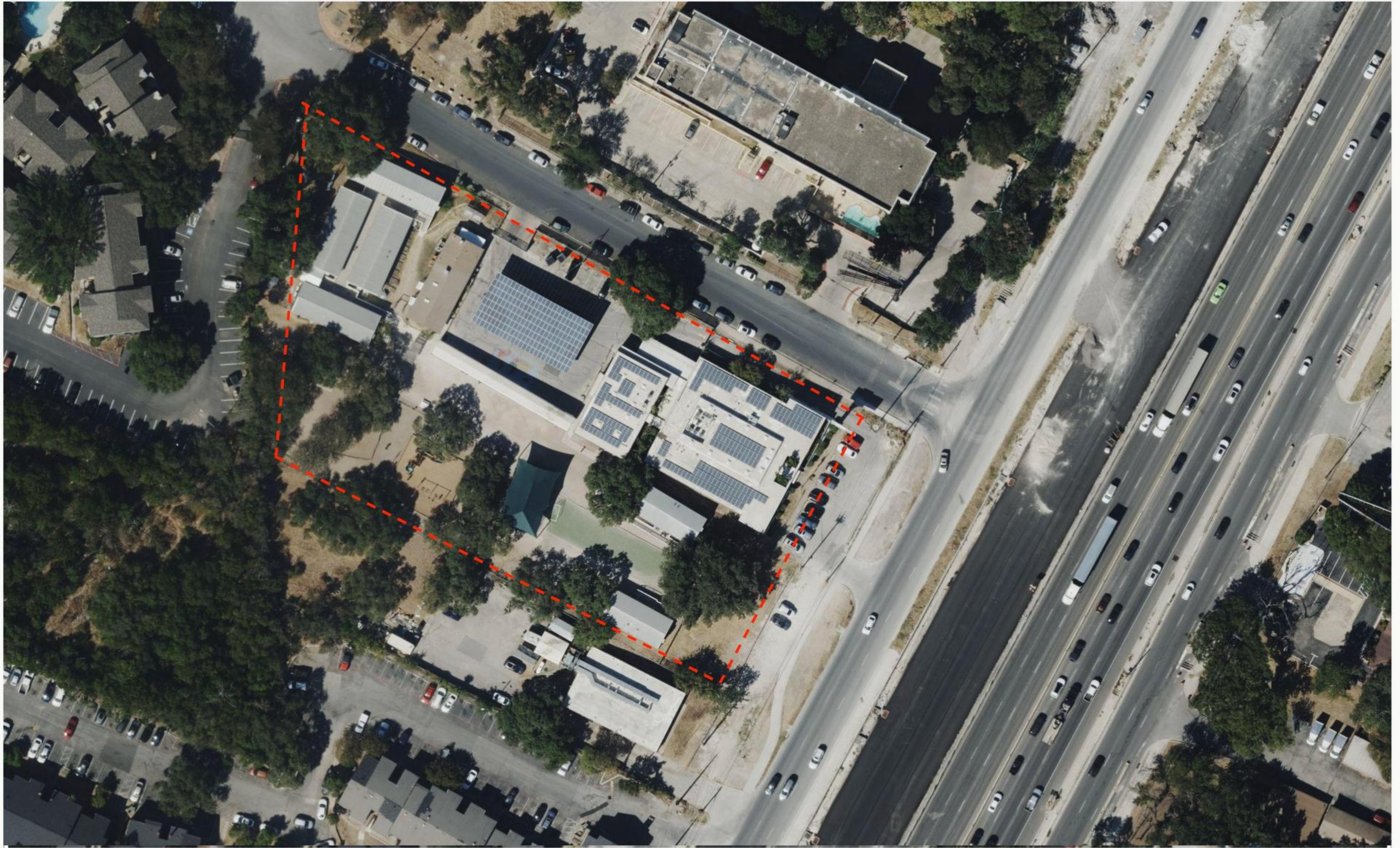
Top-down aerial — Cedars International Academy campus | Lot 1A & Lot 2A on Barwood Park, fronting I-35 SBFR
