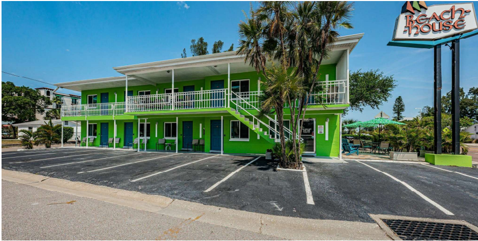
B Beach House Hotel 12100 Gulf Blvd Treasure Island, FL 33706
