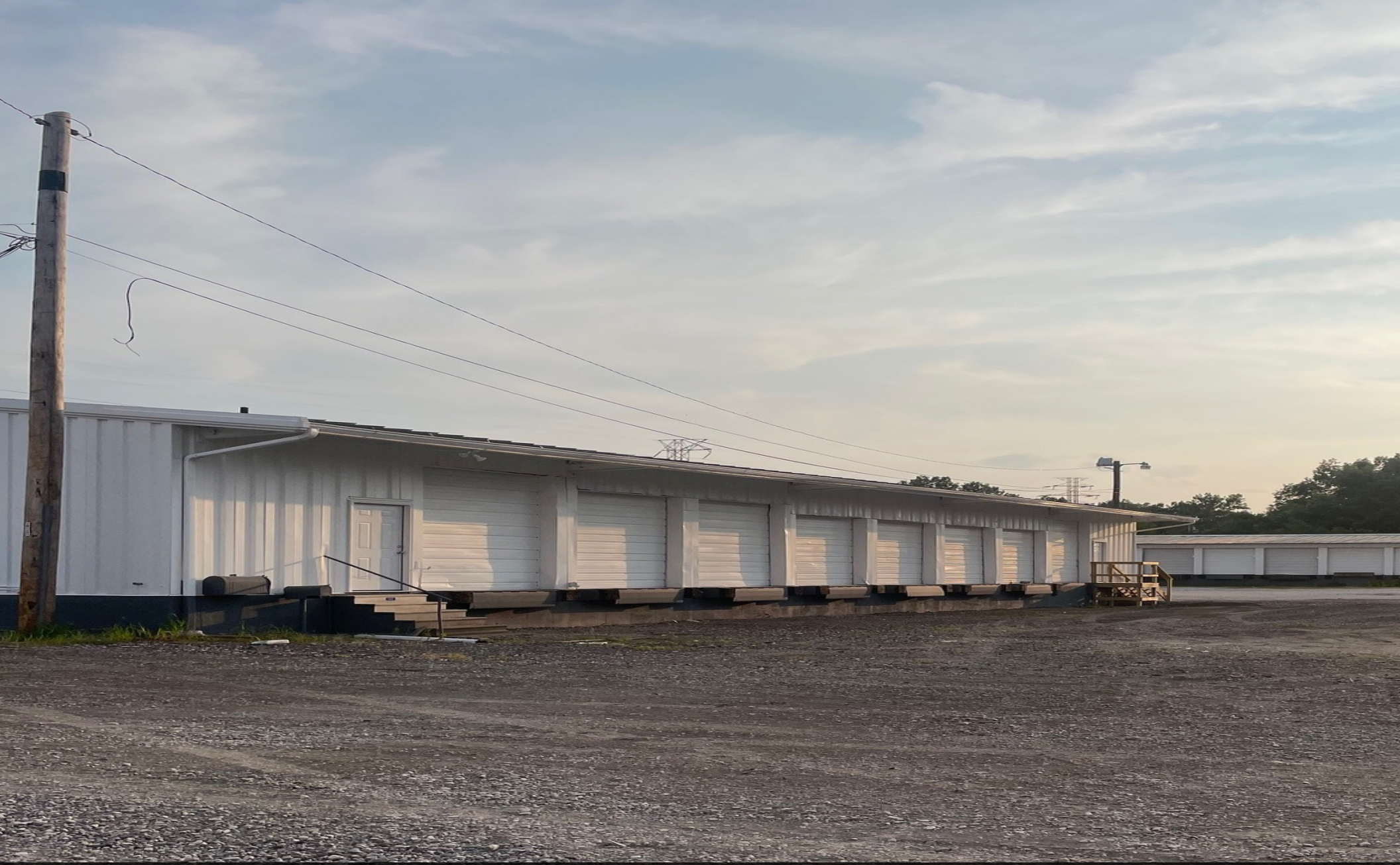
2780 Kratzville Building - 16 Door Cross Dock Terminal - Northside
