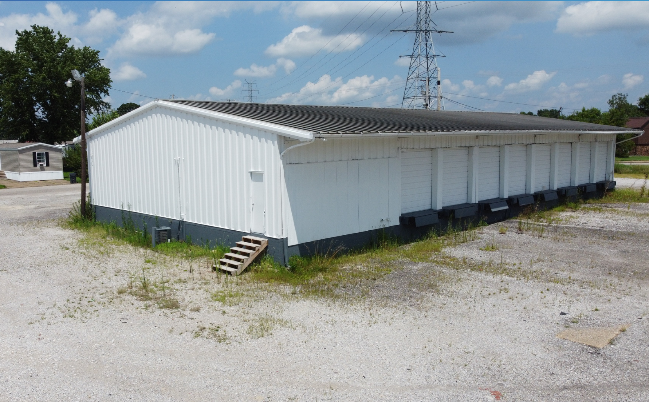
2780 Kratzville Building - 16 Door Cross Dock Terminal - Southside
