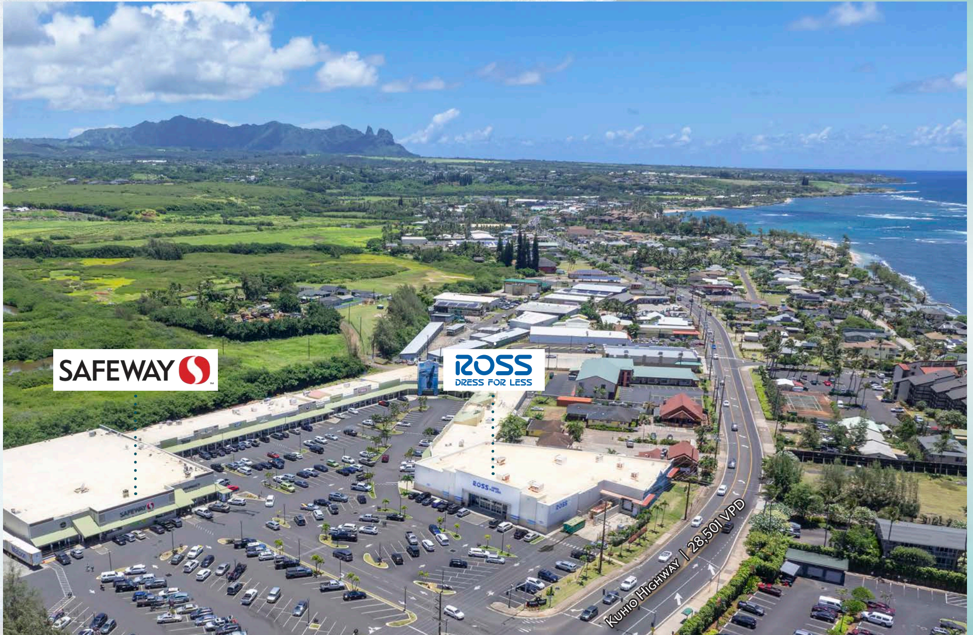
Kauai Village Shopping Center | 4-831 Kuhio Highway Kapaa, HI 96746
