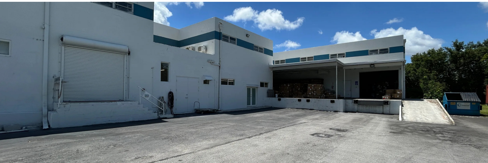
Truck Court & Front Loading Dock & Ramp
