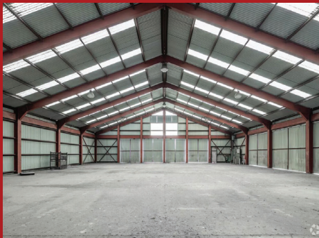
INSIDE REAR BUILDING
