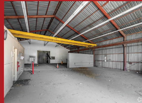
INSIDE FRONT BUILDING
