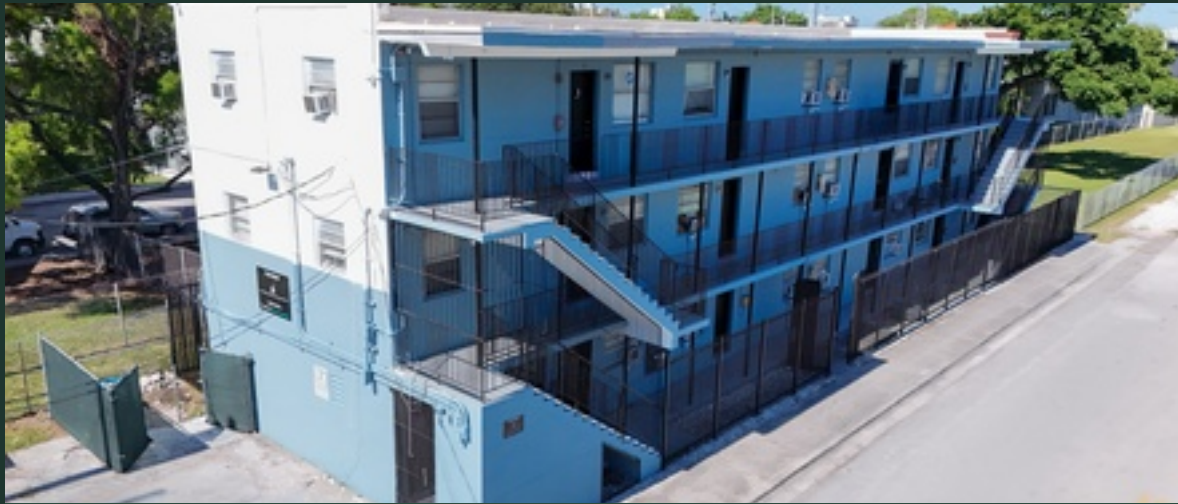
Building with Skyline Backdrop
