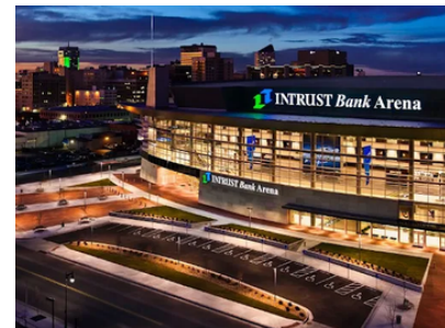
INTRUST Bank Arena
