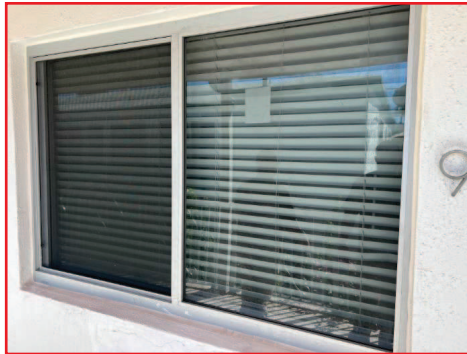
Impact Windows Noted
