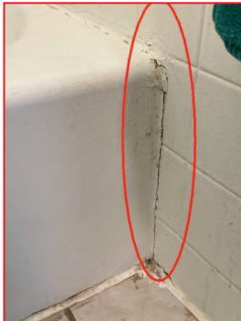
Tub needs sealing
