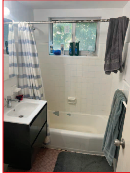
Master Bathroom View
