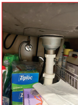
Under Kitchen Sink
