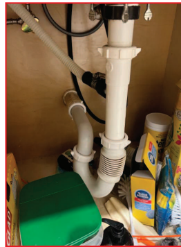
Under Kitchen Sink
