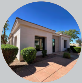
EXTERIOR LOADED ENTRY (2 POINTS)
