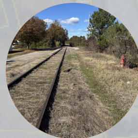
Rail Siding Adjacent
