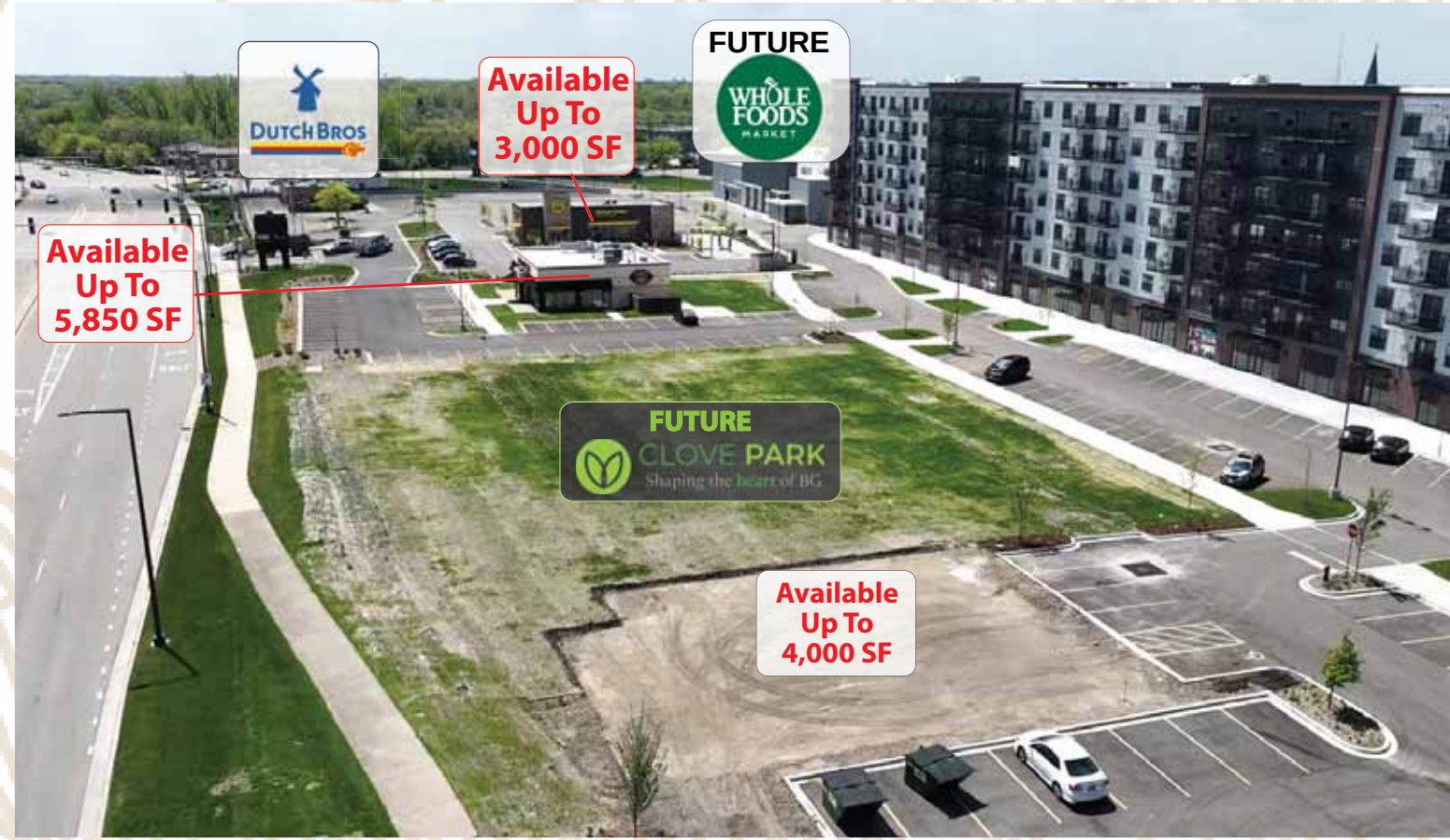
AVAILABLE BUILD-TO-SUIT PADS ON FUTURE CLOVE PARK
