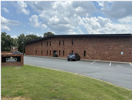
Exterior & monument signage Brick frontage, monument sign at street
