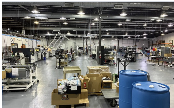
Production floor Conditioned throughout, sealed floors, overhead power and air distribution
