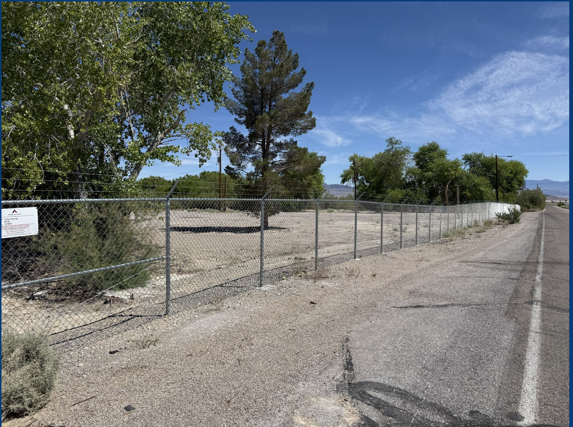
FRONTAGE FENCE – LOOKING SOUTHEAST
