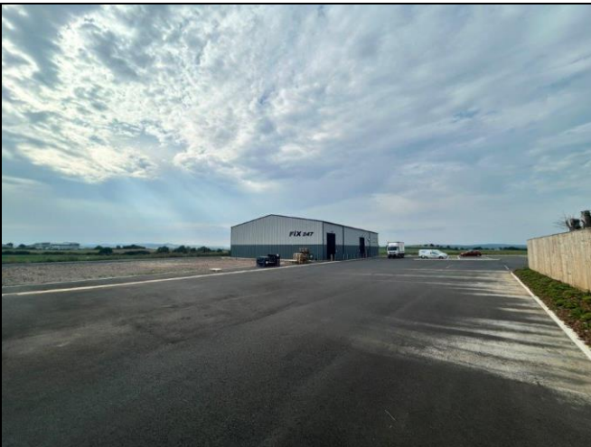
Newly built buiding at Harrier Court
