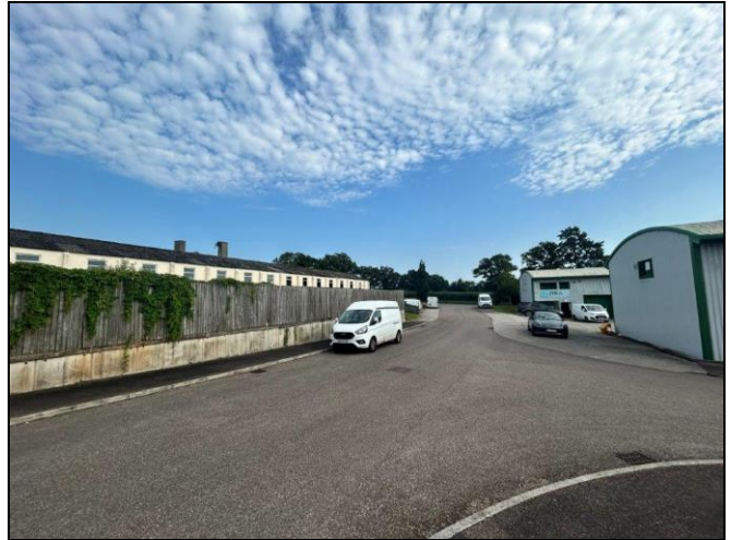
Boundary facing Harrier Court
