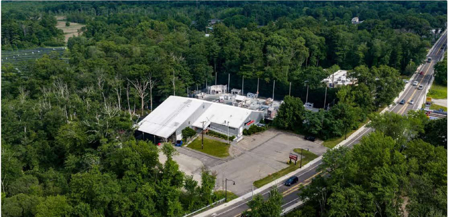
Aerial — 120 Pond Street in the Route 126 corridor
