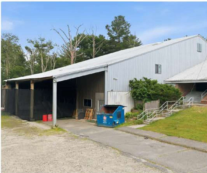
Covered grade-level drive-in loading
