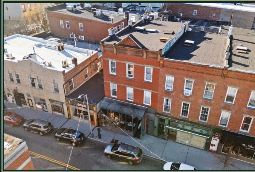
Aerial View — 8 North Broadway & Downtown Nyack Corridor
