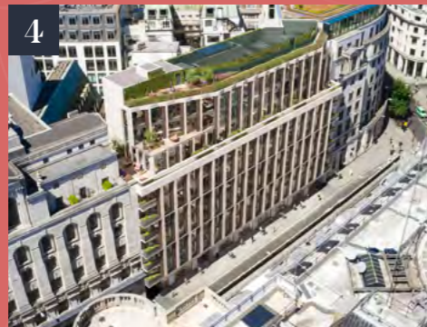
7 PRINCES STREET Developer KanAm Area 54,000 sq ft Status Completed 2025
