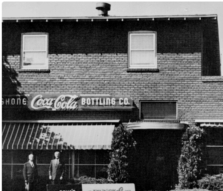
Historic Shoshone Coca-Cola Bottling Co. plant.
