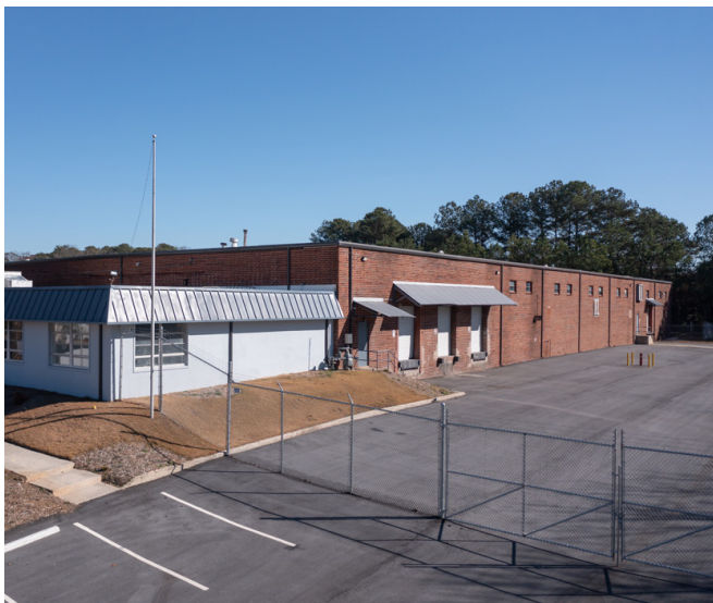
NEW SECURITY GATE AND SURVEILLANCE SYSTEM
