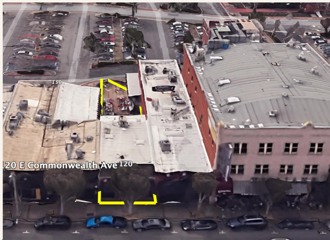
Aerial view — 120/122 E Commonwealth Ave, one block west of S Harbor Blvd
