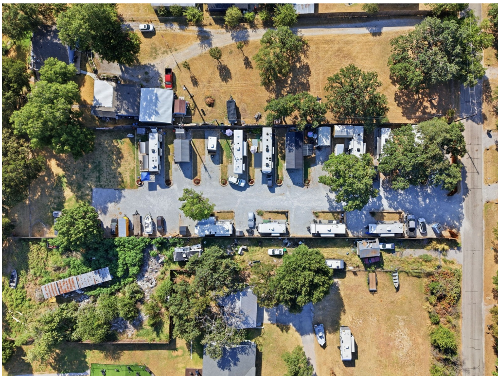
Aerial overview of the RV pad layout and internal drive.
