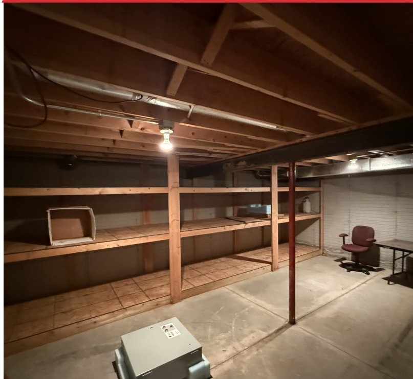
Basement Of Office Area
