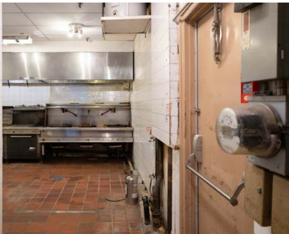
Dedicated loading and delivery door
