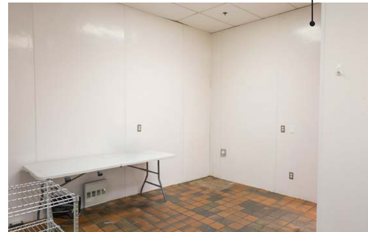
Backroom for food preparation and storage
