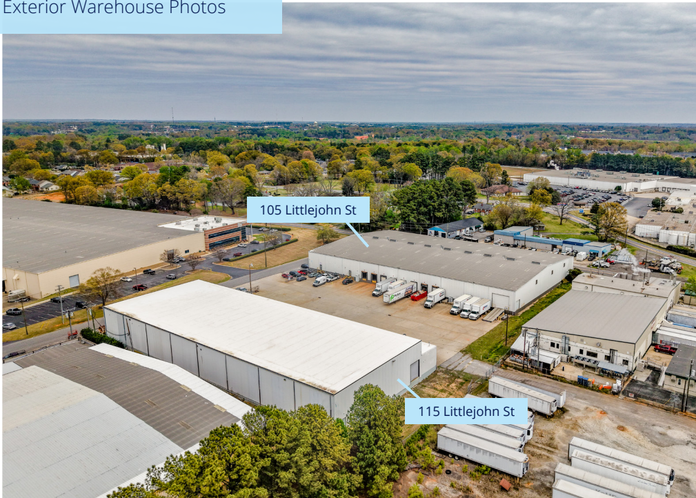
Exterior Warehouse Photos
