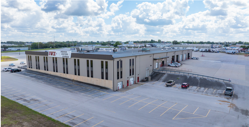
Northwest Side of Property
