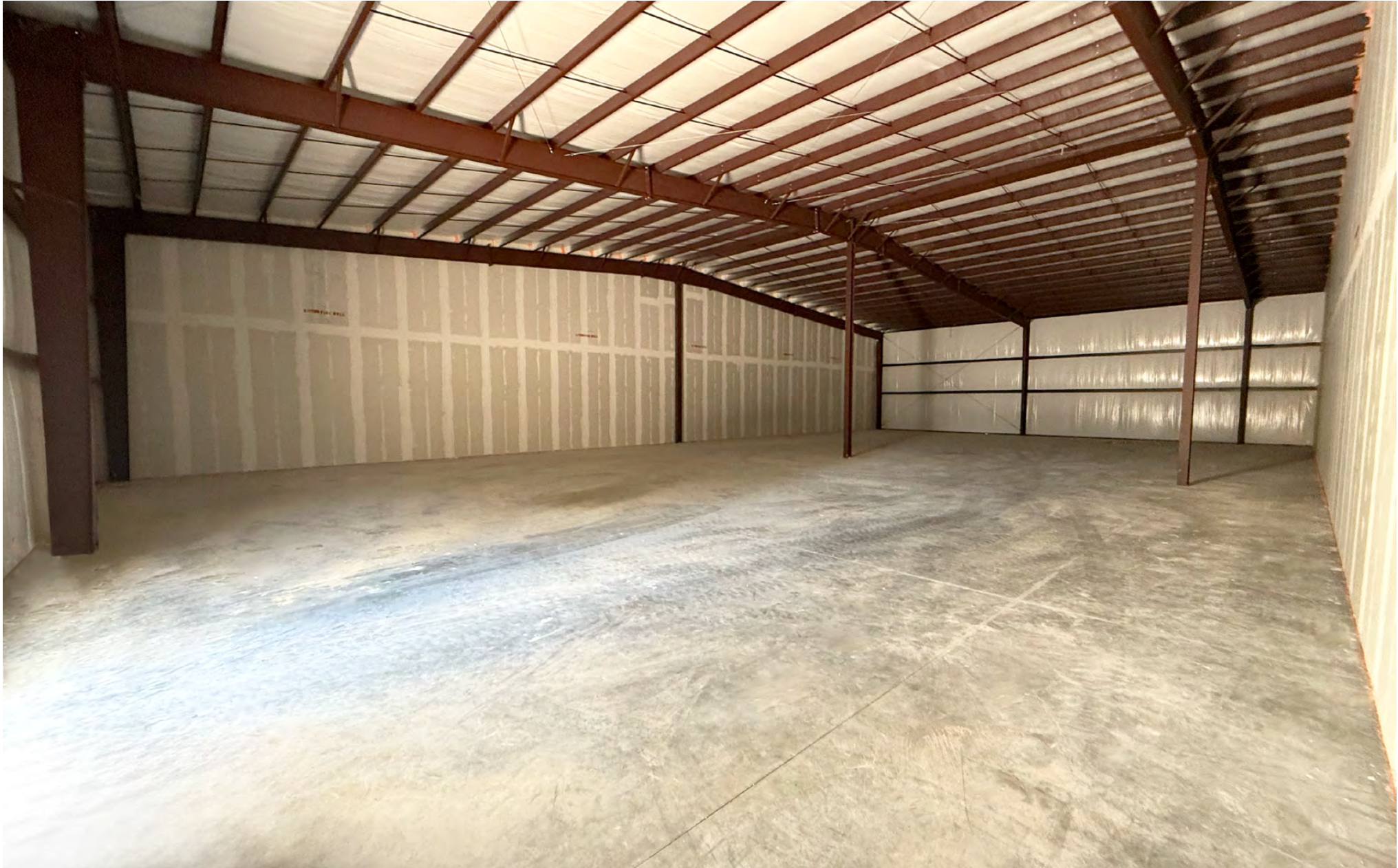
Interior Spaces Construction Progression September 2025
