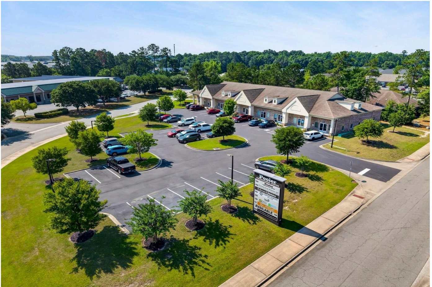
Pooler Professional Center (foreground) with Pooler Pkwy commercial corridor visible — tenant directory includes Suite 101 (available), Edward Jones, Pooler Family Medicine, Surge Staffing and others
