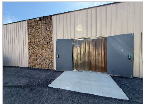
Rear service access
