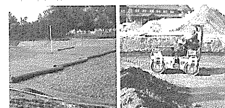
Install non-woven geotextile over stone. Geotextile must overlap 24" (600 mm) min. where edges meet. Compact each lift of basefill as specified in the site design engineer's drawings. Roller travel parallel with rows.
