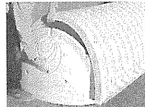
Lift the end of the chamber 3" from the ground. With the curved face of the end cap facing outward, place the end cap into the chamber and compress.
