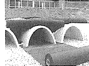
Place a strip of ADS non-woven geotextile over the row of chambers (not required over DC-780). This is the same type of non-woven geotextile used as a separation layer around the angular stone of the StormTech system.
