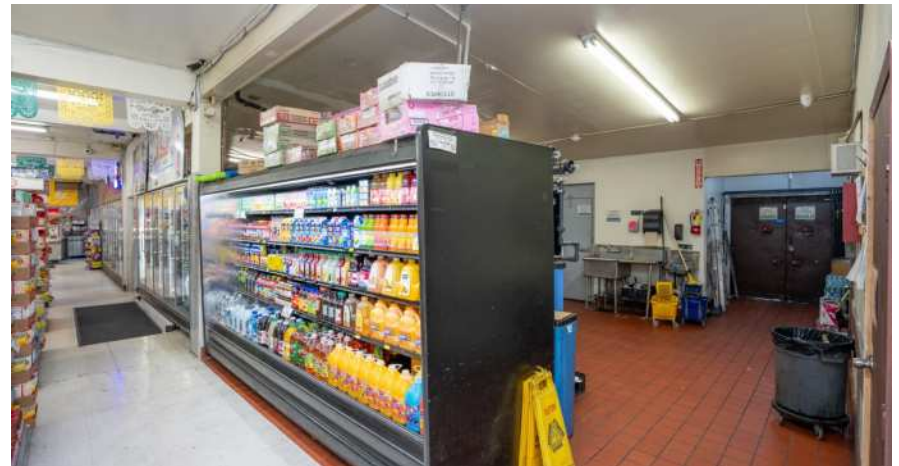
COOLERS / OPERATIONS AREA
