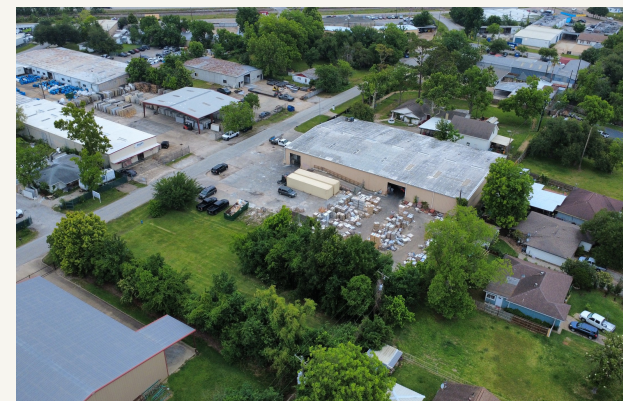
AERIAL — LOOKING EAST
