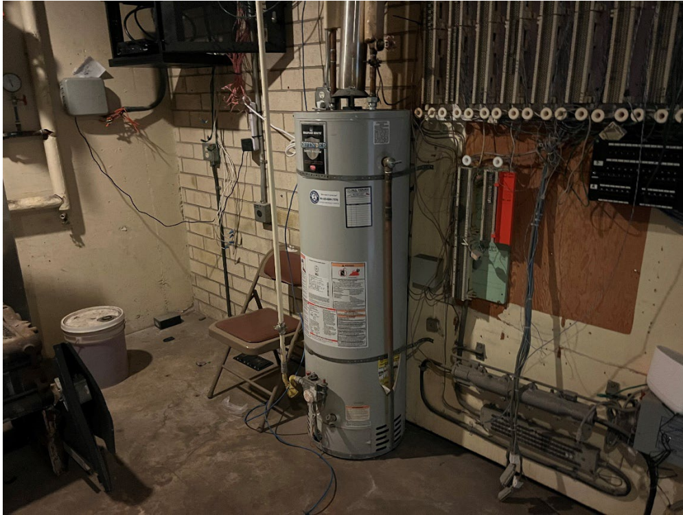
Photo 7 - View of the water heater, which is located in the basement.
