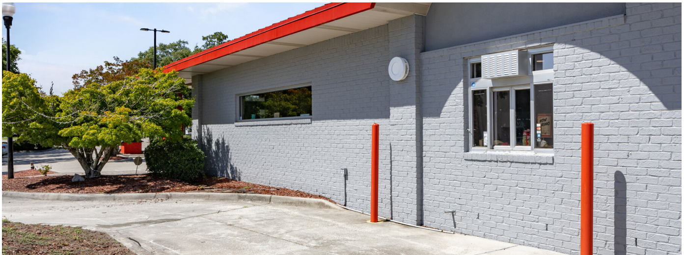
Rear and side building elevation, showing the signature red standing seam roofline, painted brick exterior, and covered walkway.
