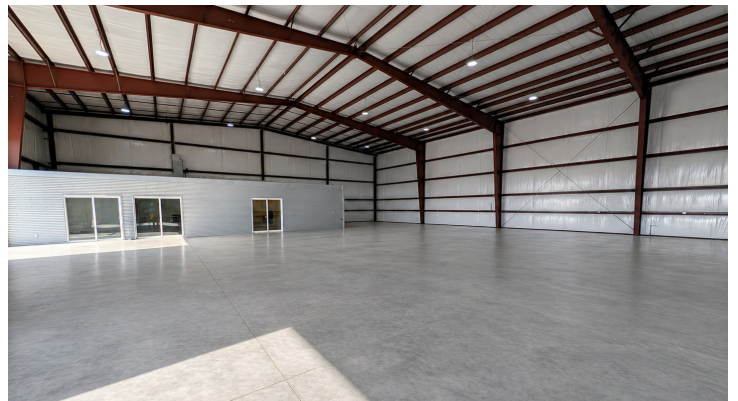
Warehouse Facing North
