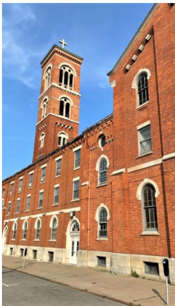
North side Allen St Bldg.
