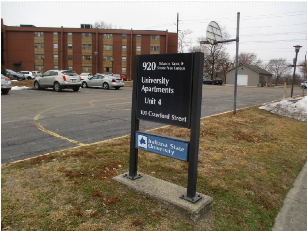
Two views of Unit 4 from Crawford Street.
