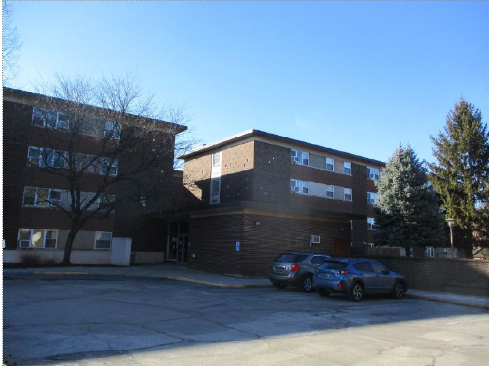
The centrally located entry on the east side of Unit 1. The north wing for Unit extends to the right side of the picture. The south wing extends to the left side of the picture.
