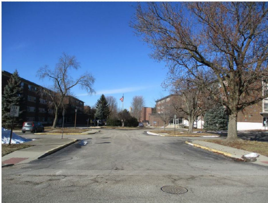
north view from Farrington Street along the driveway that extends to a cul-de-sac between Units 1 and 2. Unit 1 is to the left side of the picture. Unit 2 is to the right side.
