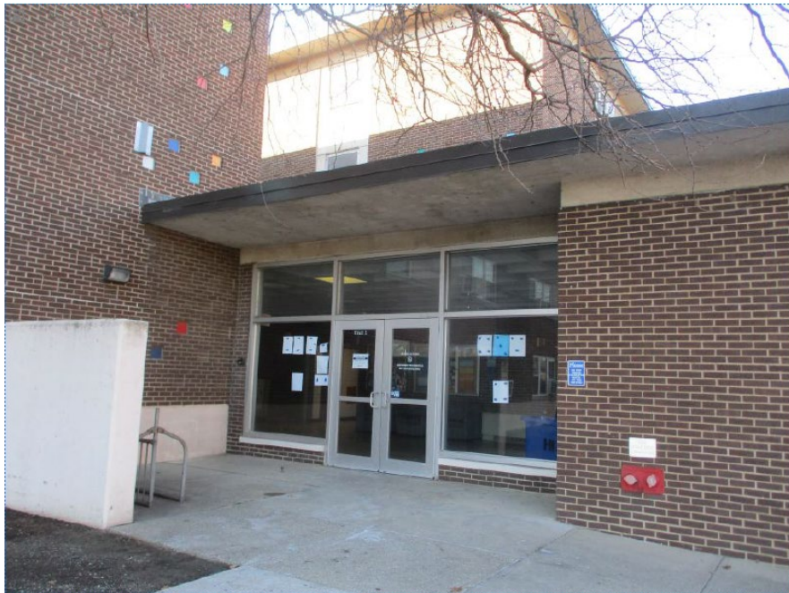
The centrally located entry on the east side of Unit 1.
