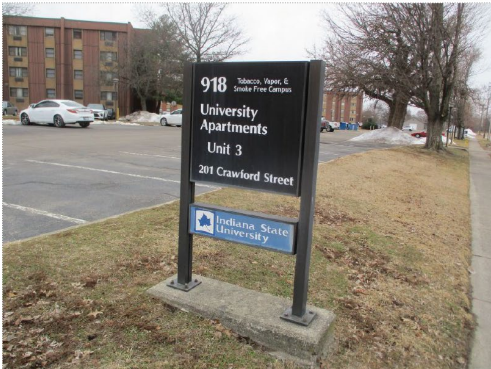
Two views of Unit 3 from Crawford Street.
