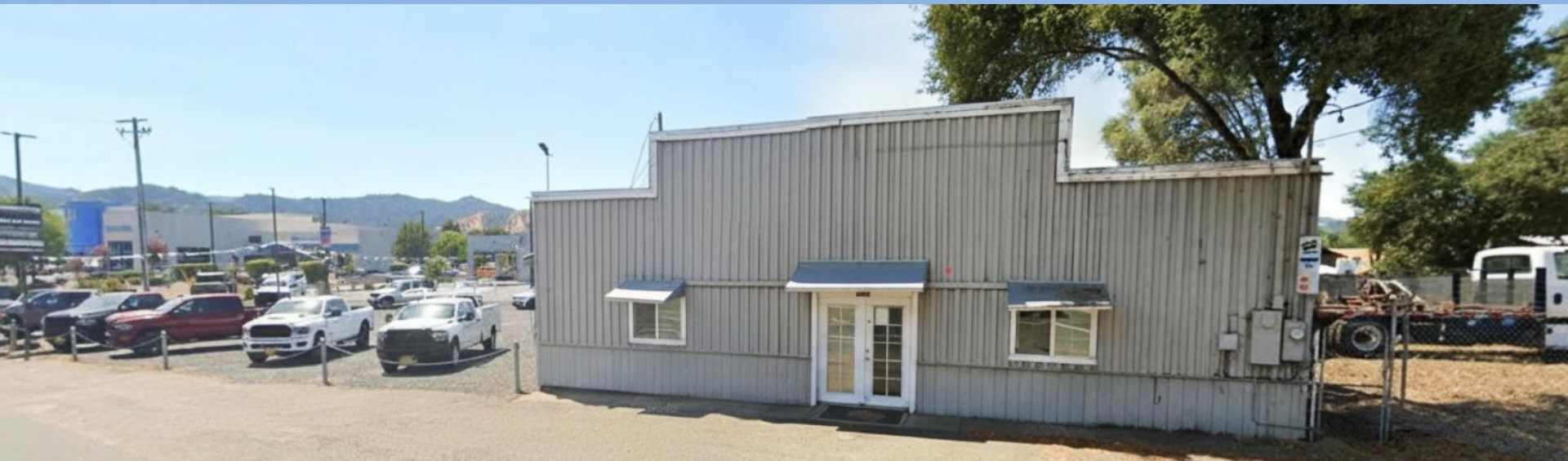
Street view: Santa Rosa Ave
