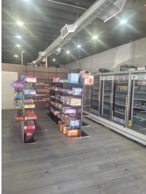
After tenant improvement
