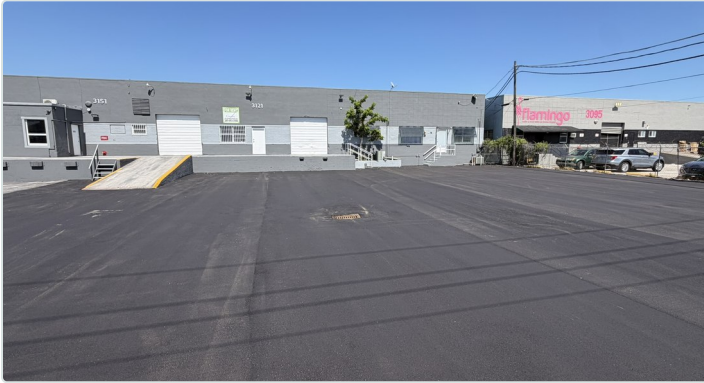
Gated Yard &amp; Dock-High Loading Ramp
